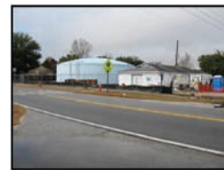
Mitchell WTP Looking Northwest
